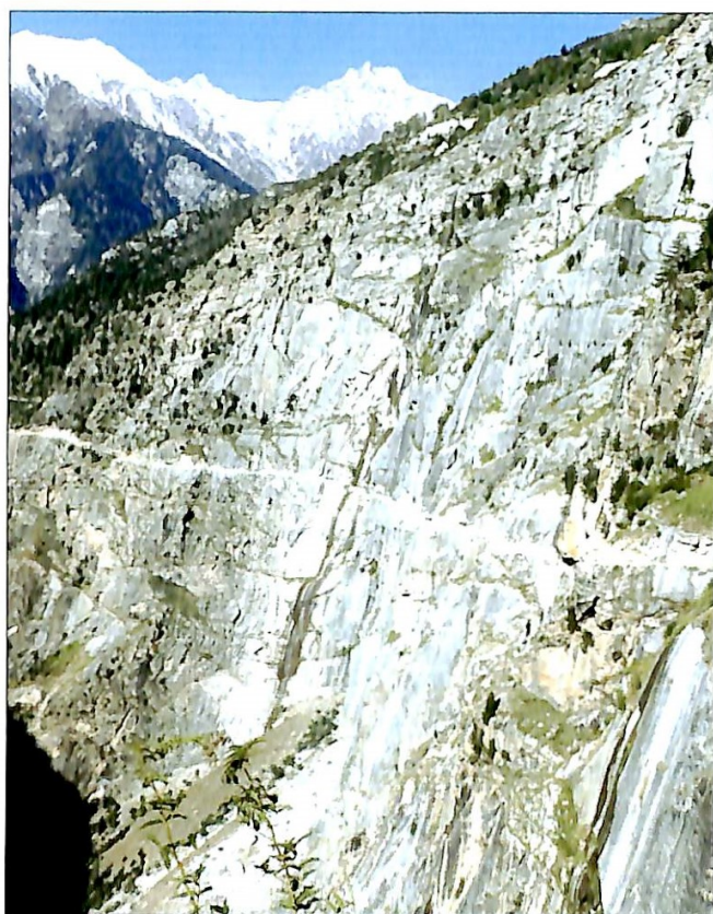
Dangerous motor road leading to Killar (Harish Kapadia)
