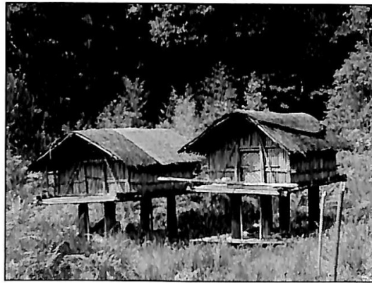
4. Raised houses to prevent rain damage. (Harish Kapadia)
