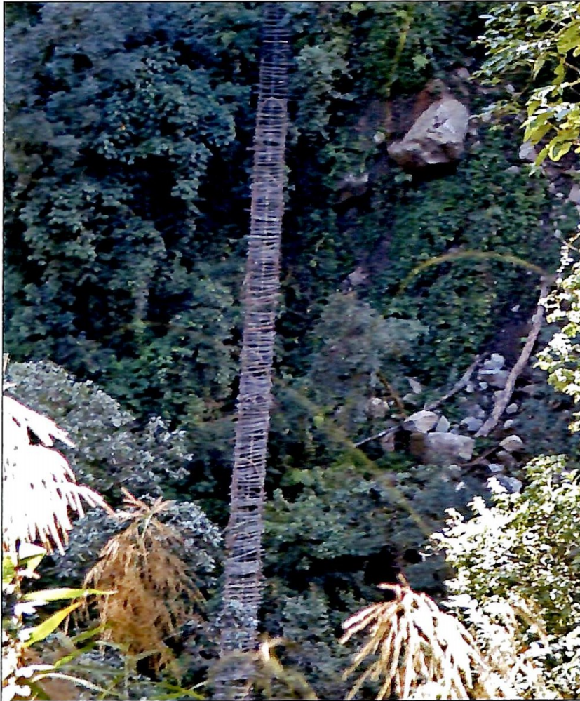
37. A long 'Foot Suspension Bridge' (FSB).
