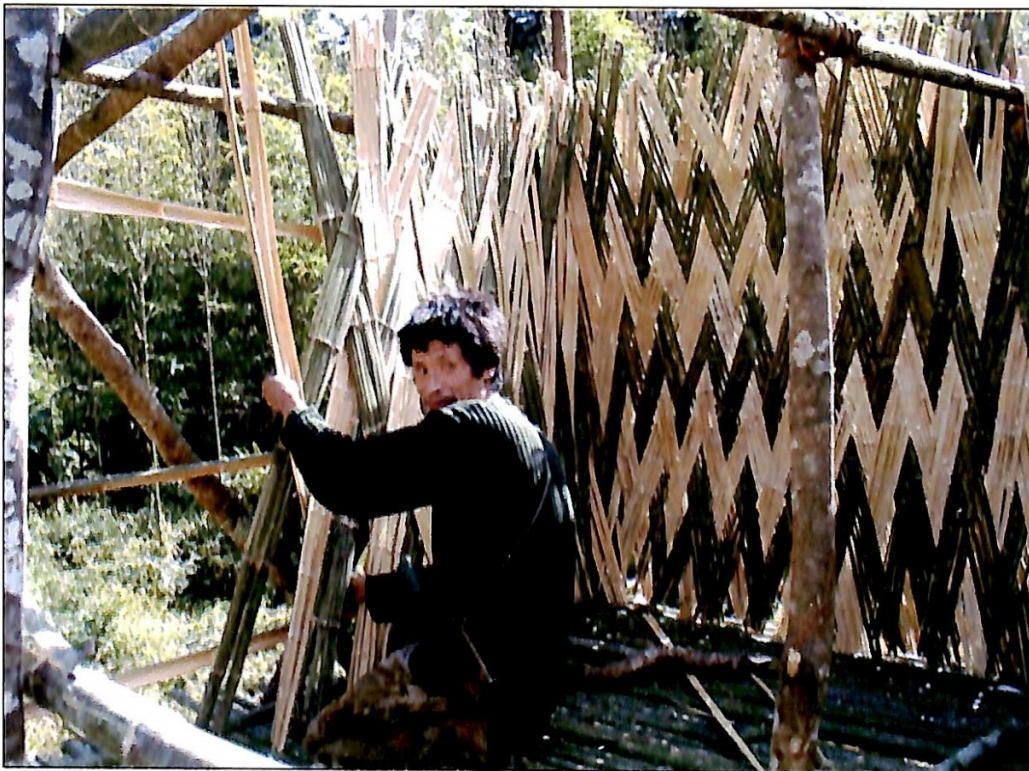
42. Erecting traditional bamboo hut.
